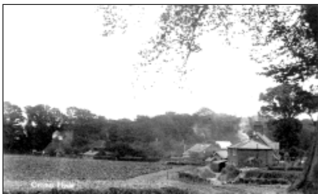
Photograph taken before the fir trees were planted
